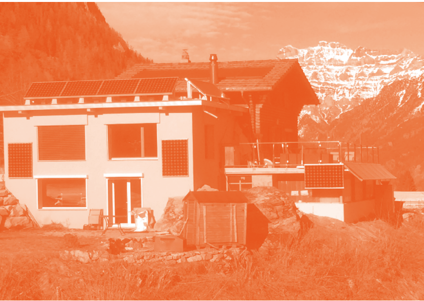
Figure 2: Switzerland, Les Marécottes, unfortunate solar panel installation. © Oliver Martin
